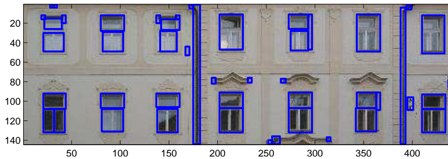
Figure 4: The result of find windowpanes with external prior operator to support breaking of the windows in the lower row.
